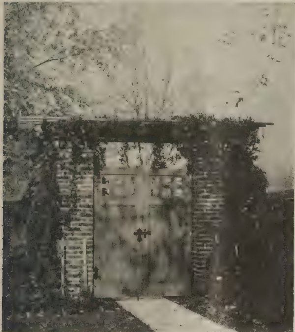
GATEWAY WITH BRICK PIERS AND LATTICE OVER TO PRODUCE A PERGOLA EFFECT.
